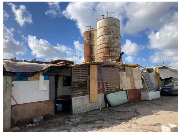
The former accommodation of seasonal workers in Campobello di Mazara, photo: borderline-europe
