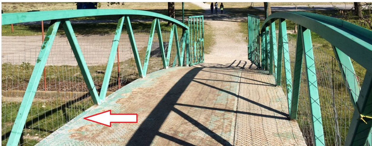
Flimsy fencing which comes away from the bridge deck/floor
